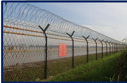
Fencing at Punggol Barat
